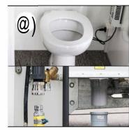
Empty toilets by flushing them one last time. Then disconnect the drain.
