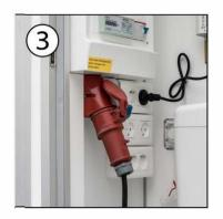
Connect the electrical cable and switch on all switches. If the trailer has waste disposal, connect it and switch it on.
