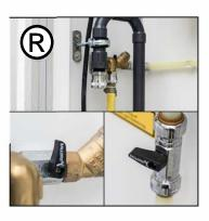
Connect the water hose and turn off all drain taps. Turn on the water and the main tap.
