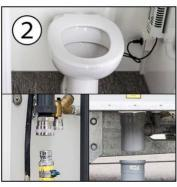
Empty toilets and cisterns by flushing them one last time. Then disconnect the drain.
