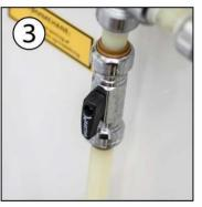
Empty the water heater and hoses by opening all the drain taps.
