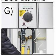
Turn off the water heater and disconnect the water supply. (It must not be switched on without water)
