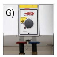
Turn off the water heater by turning the thermostat to zero. (It must not be switched on without water)
